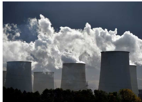
General view of the coal power plant of German LEAG energy company, in Jaenschwalde, Germany, October 21, 2021. Picture taken October 21, 2021. REUTERS/Martinus Rietchel Purchase Licensing Rights
